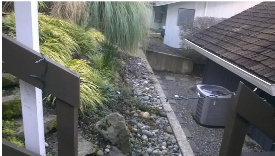
Figure 3. Area of proposed new watercourse buffer impacts. The proposed addition would extend 3 feet beyond the existing concrete retaining wall.
